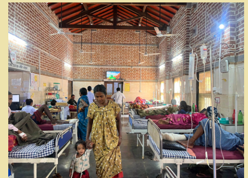
High roof wards ensuring adequate ventilation and lighting
